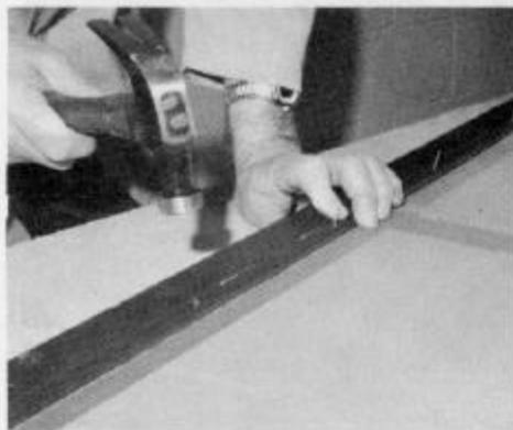
Step 9. Replace the wood strips around each panel. If they were broken when removed, you may have to buy new ones. Paint the entire frame. Keep screen frames painted. When the paint peels off, moisture gets into the wood. This can cause the frame to swell and will eventually cause the frame to rot.
